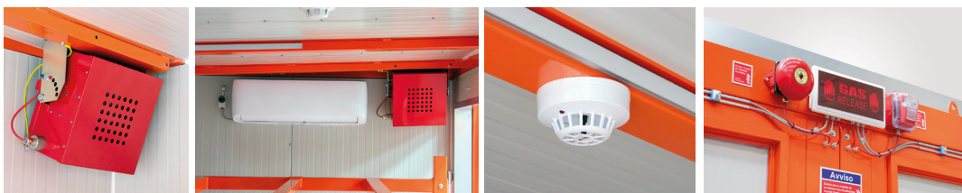
Concentrated aerosol fire suppression system - KIWA certified
